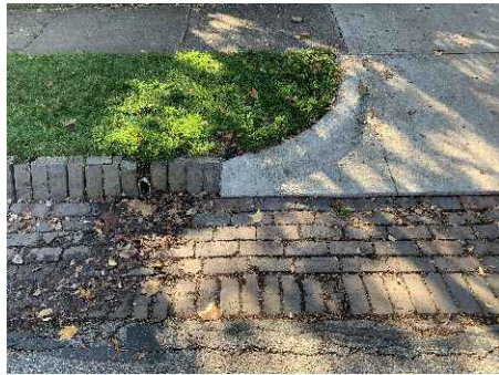
ACCEPTABLE CONCRETE APRON RETURNS TO EXISTING BRICK CURB AND GUTTER
