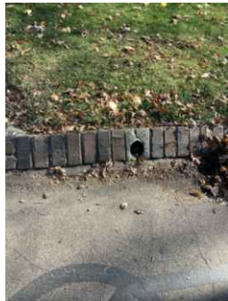
ACCEPTABLE DRAIN PIPE THROUGH BRICK CURB
