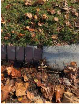
ACCEPTABLE CONCRETE APRON RETURNS TO EXISTING BRICK CURB
