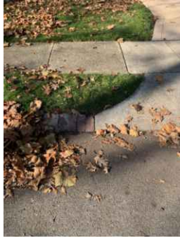
ACCEPTABLE CONCRETE APRON RETURNS TO EXISTING BRICK CURB
