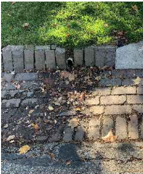
ACCEPTABLE DRAIN PIPE THROUGH BRICK CURB
