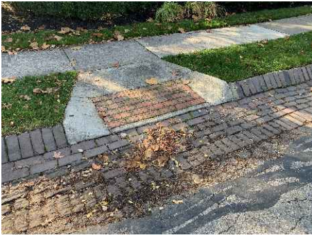
ACCEPTABLE CONCRETE APRON RETURNS TO EXISTING BRICK CURB AND GUTTER
