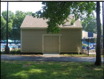
Pool Mechanical Building (n)
