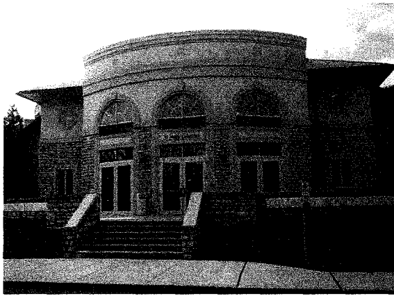
Photo C7: Classroom Building – NE entry
