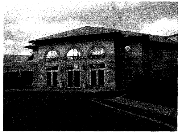
Photo C8: Classroom Building – SE entry
