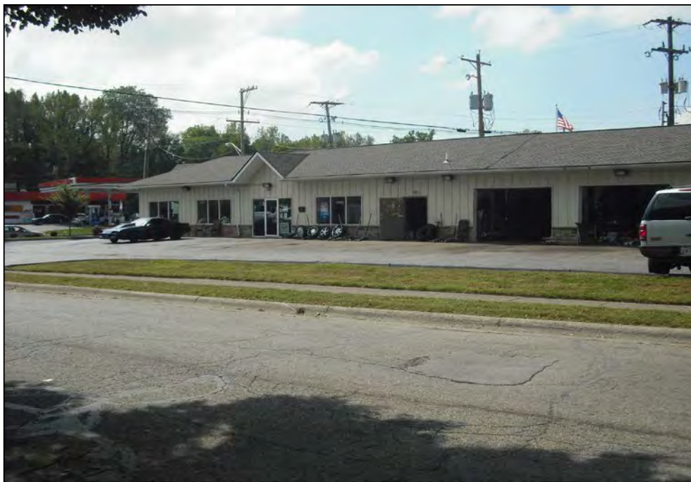
View west of Katz Tire located across Mayfield Place from the on-site multi-family residences.
