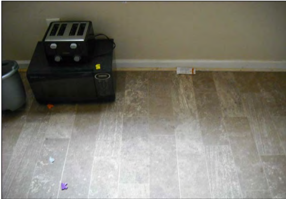
Laminate floor on the ground floor / basement unit of the 945 unit.
