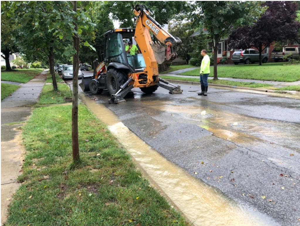
Service Department workers work a Sunday water main break on Grandon
