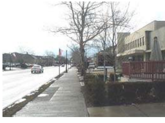
Existing Condition 'E'
