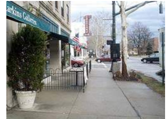
Existing Condition 'C-1'
