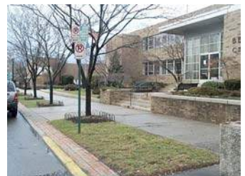
Existing Condition 'C-3'
