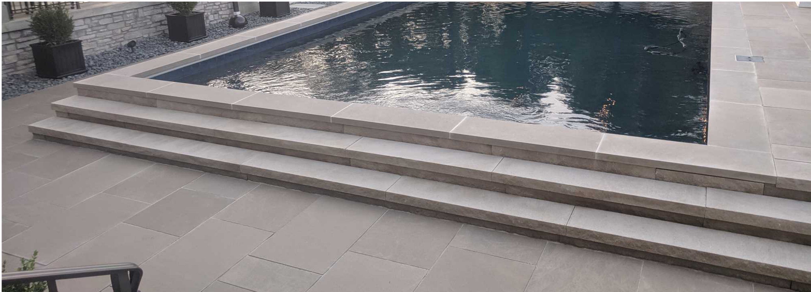
INDIANA LIMESTONE | POOL COPING, STEP TREADS AND RISERS, ALL WALKWAYS AND PATIO SURFACES
