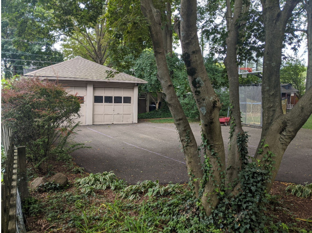
View of Garage from NW Corner of Backyard
