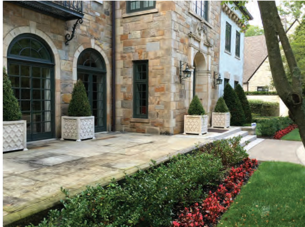
1. SANDSTONE QUOINS AND GRANITE WALL STONE
