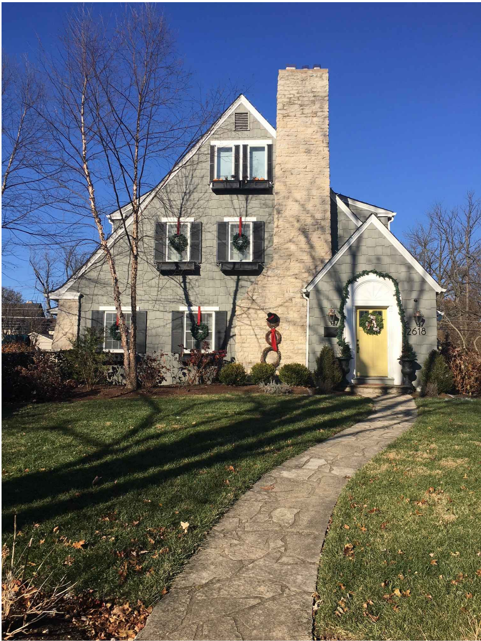
EXISTING SOUTH FACADE
