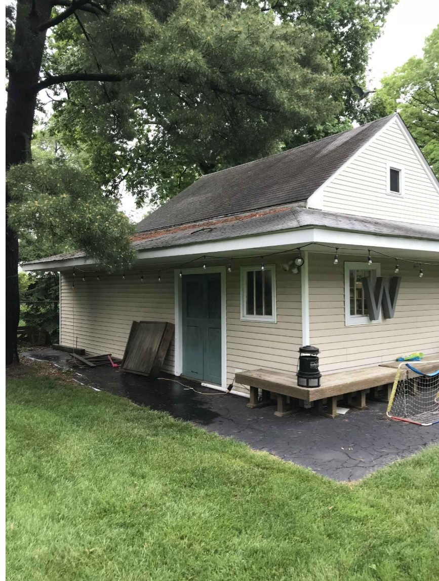
SOUTH WEST CORNER OF GARAGE
