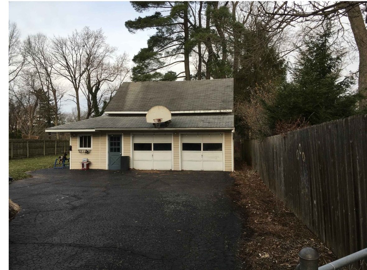
EAST FACADE OF GARAGE
