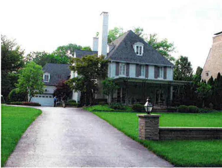
Photos of Existing West Side of Residence
