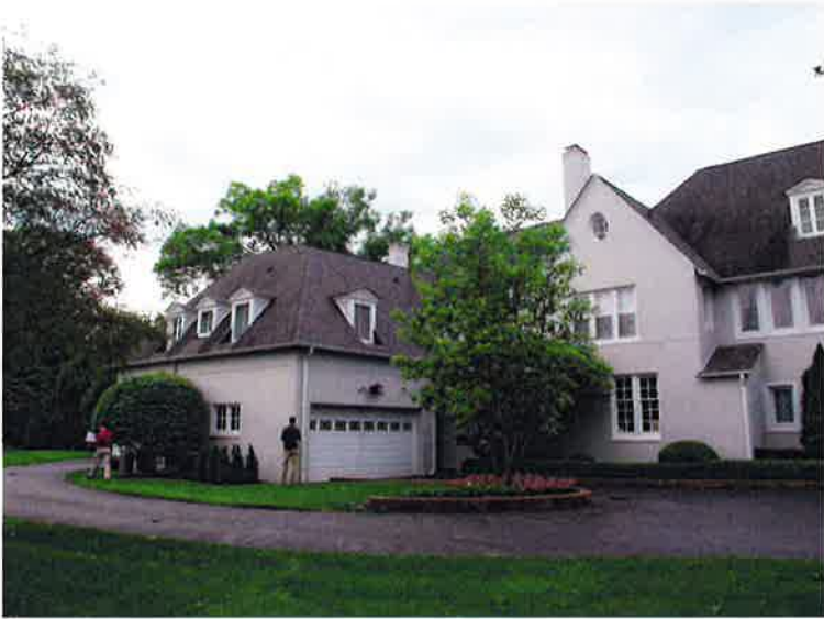
Photos of Existing North Side of Residence
