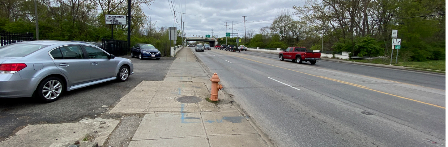
Unsafe pedestrian/sidewalk conditions
