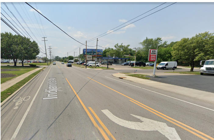
Parsons Ave Road Diet
