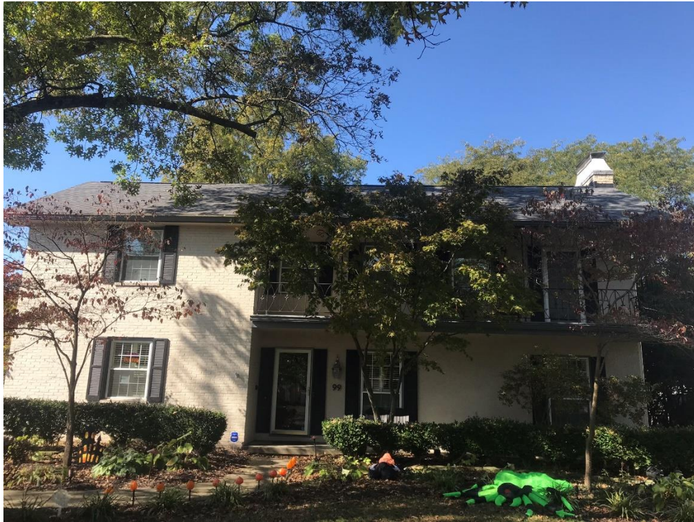
Front (East) Side
