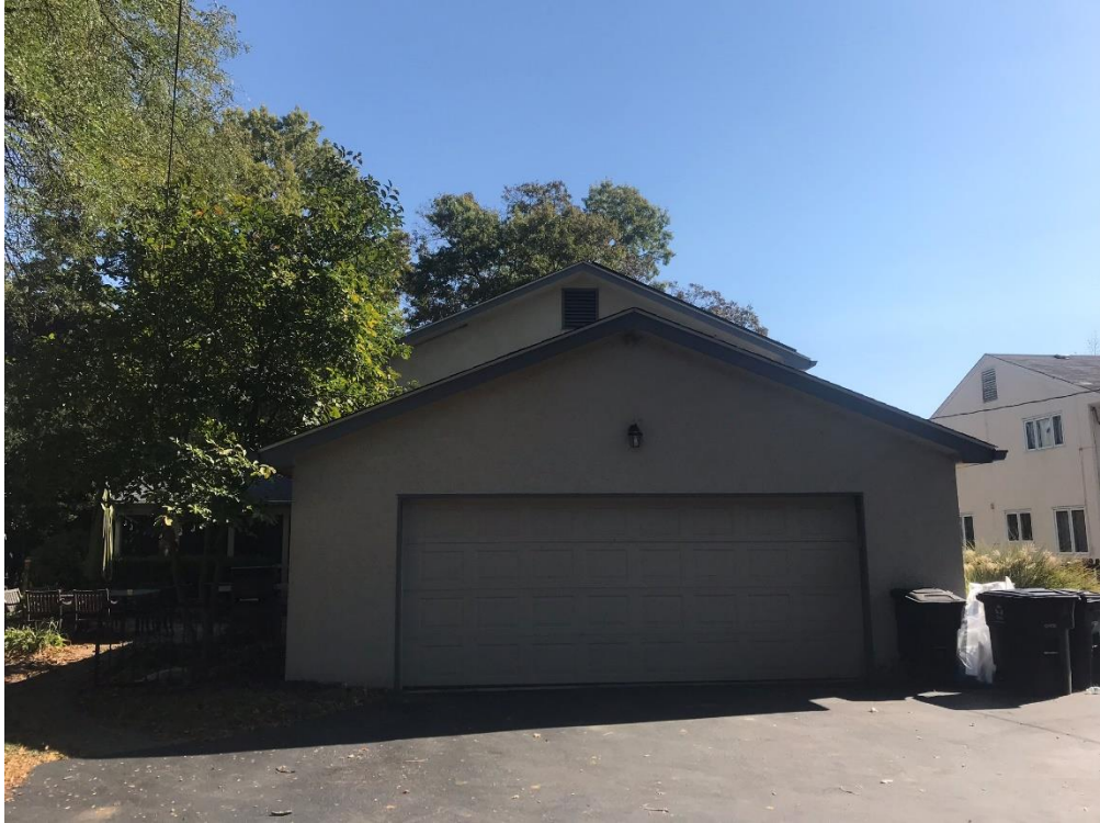
Rear (West) Side
