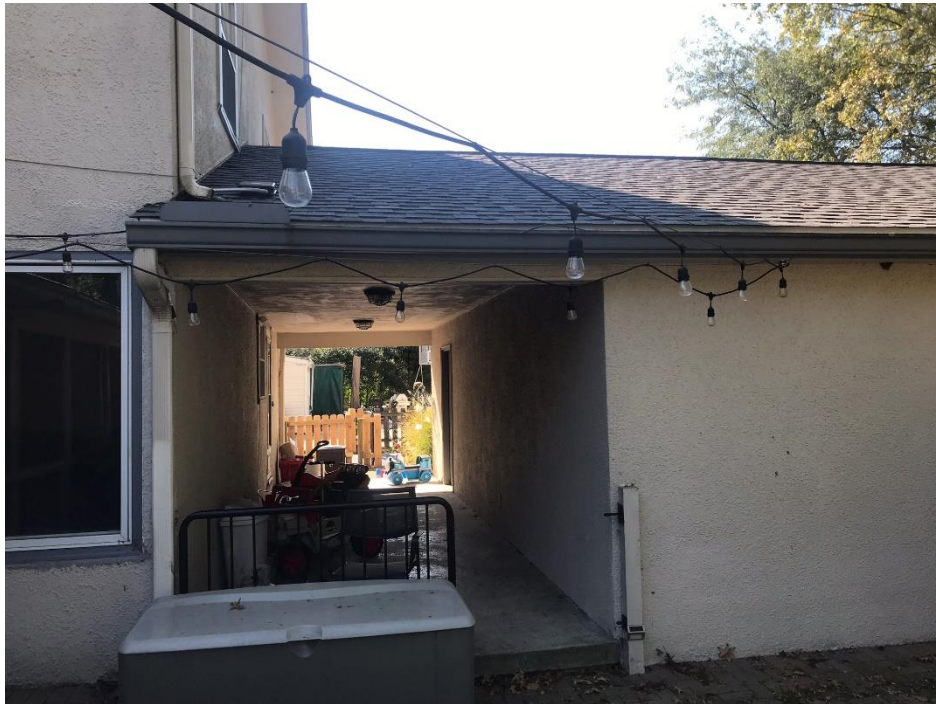
Right (North) Side – Enclosure Location
