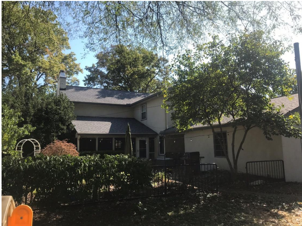
Rear (West) Side
