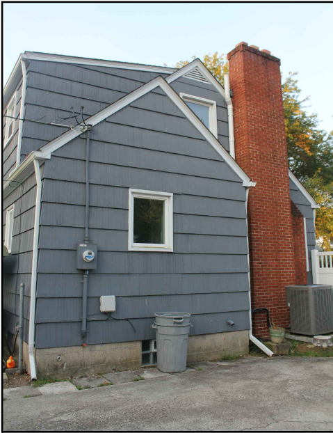
Photo of Existing North Side of Residence
