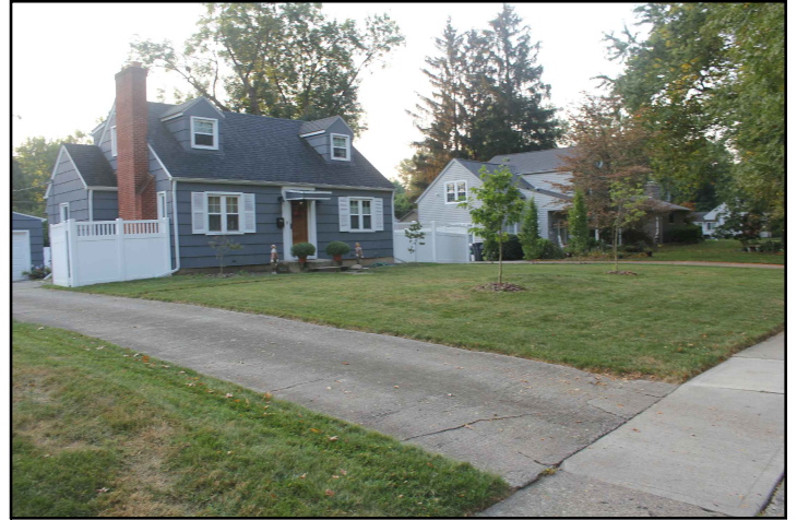
Photo of Existing West Side of Residence
