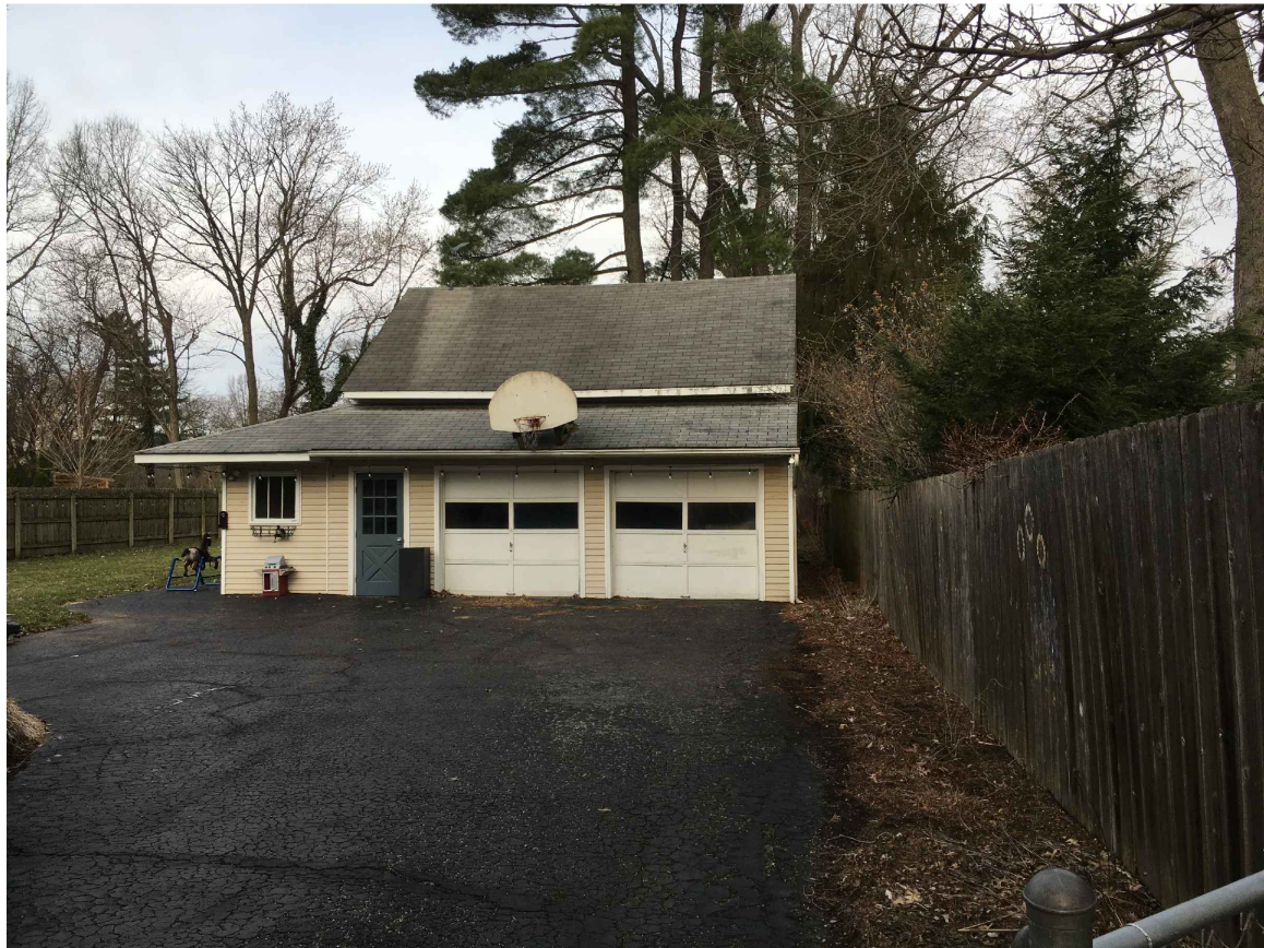
EAST FACADE OF GARAGE
