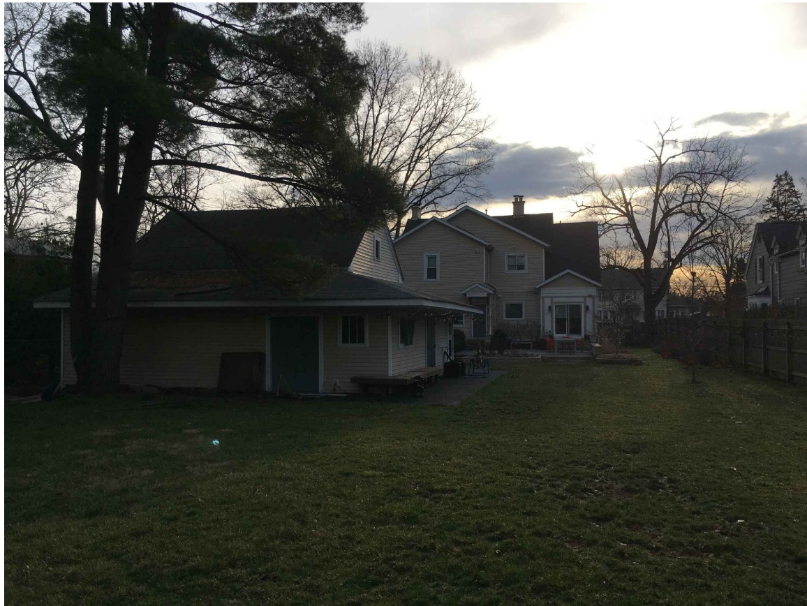
SOUTH FACADE OF GARAGE
