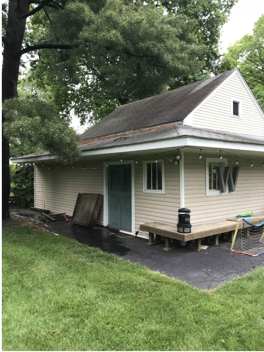
SOUTH WEST CORNER OF GARAGE
