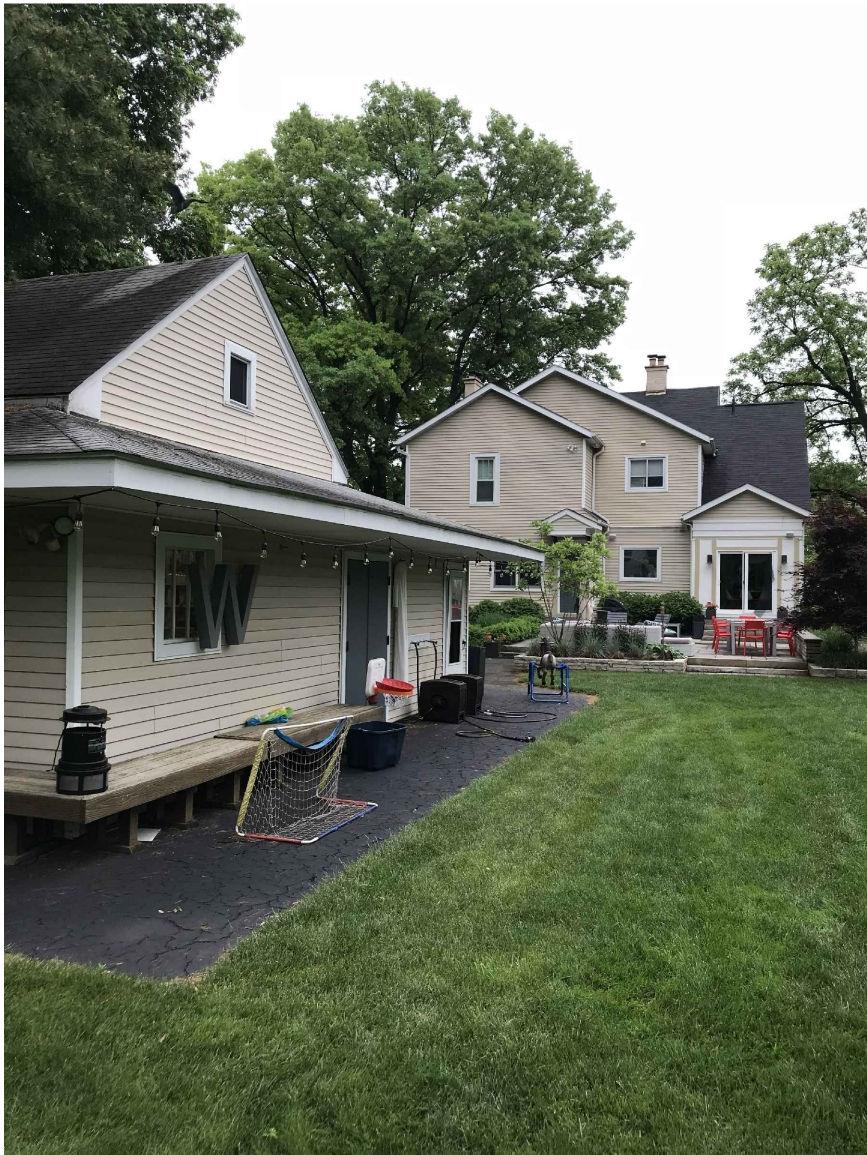
WEST FACADE OF GARAGE/ SOUTH FACADE OF HOUSE
