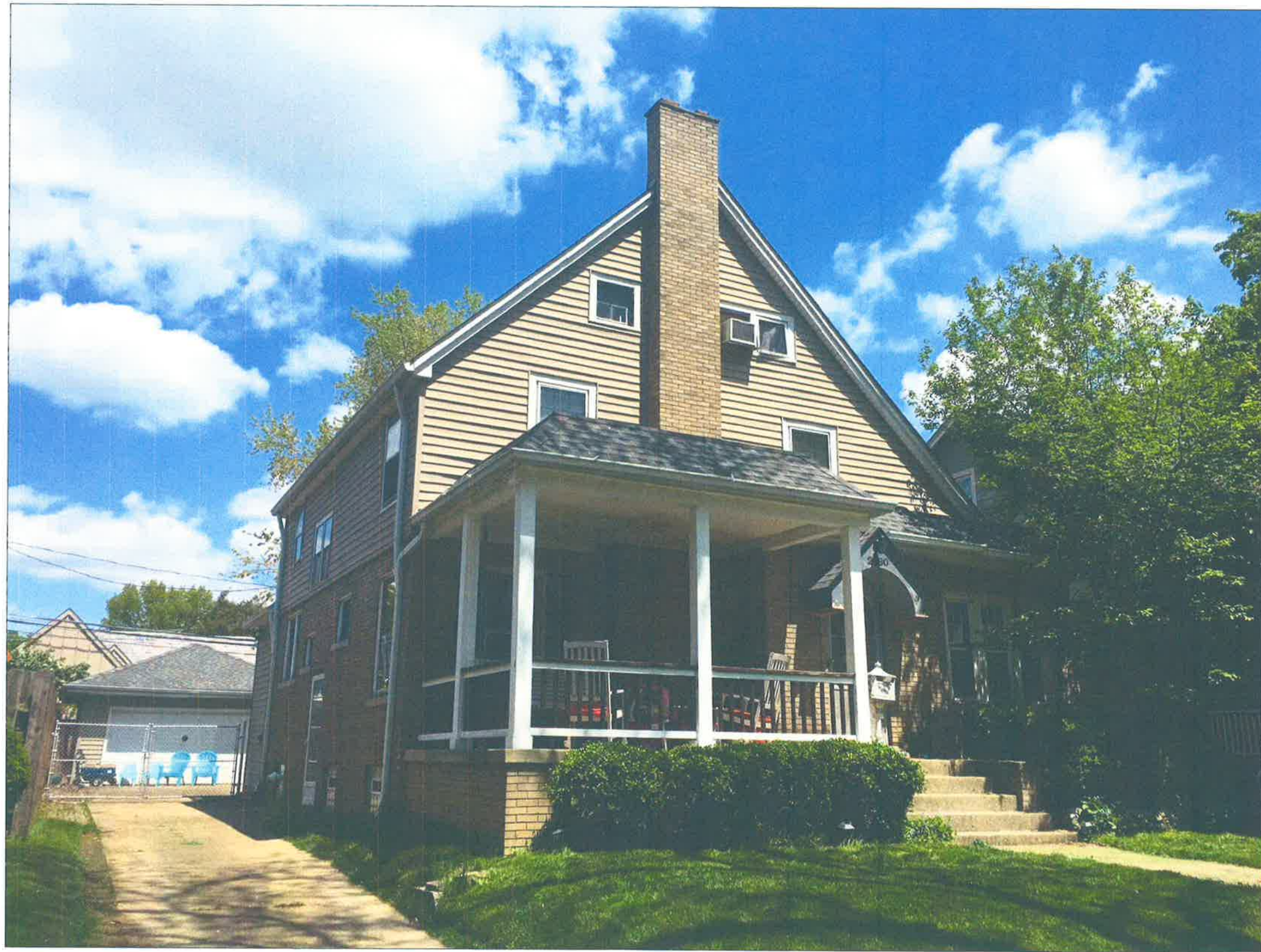
FRONT FROM SOUTHWEST
