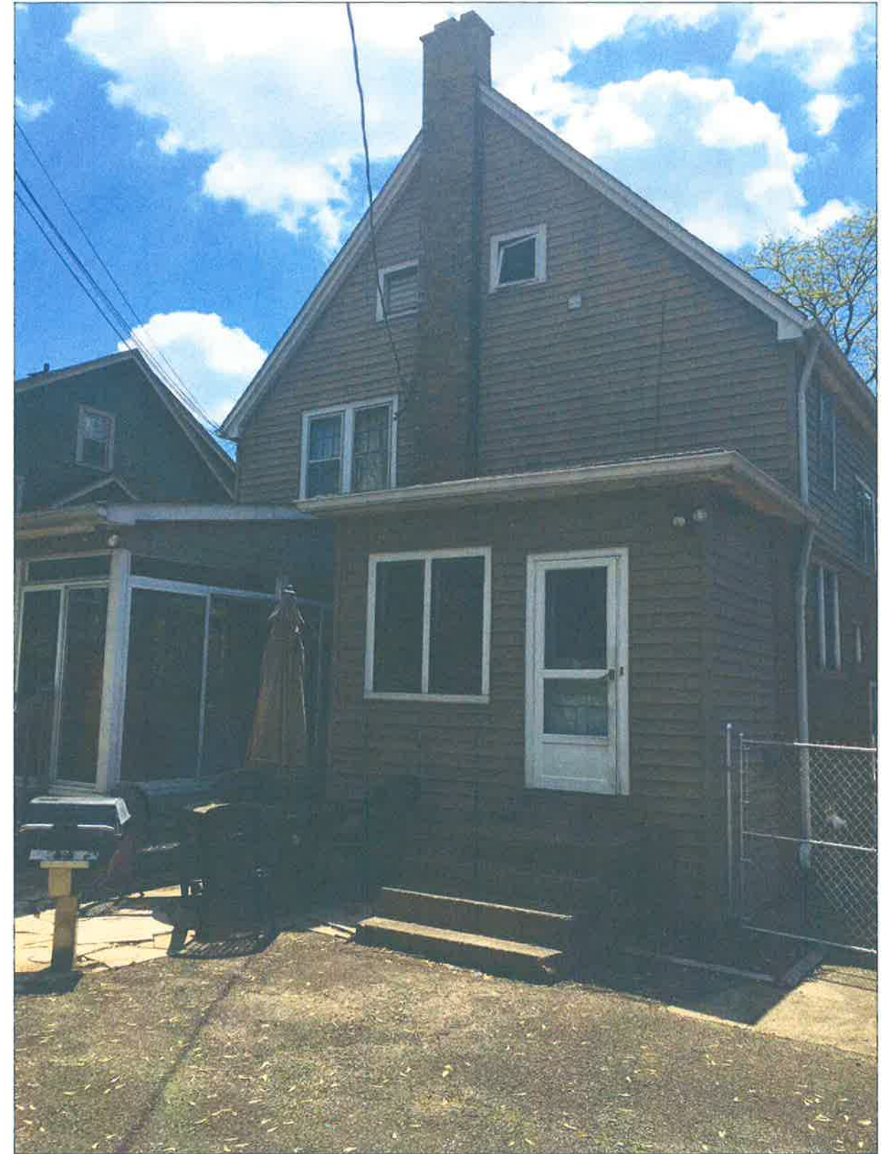
REAR FROM NORTHWEST
