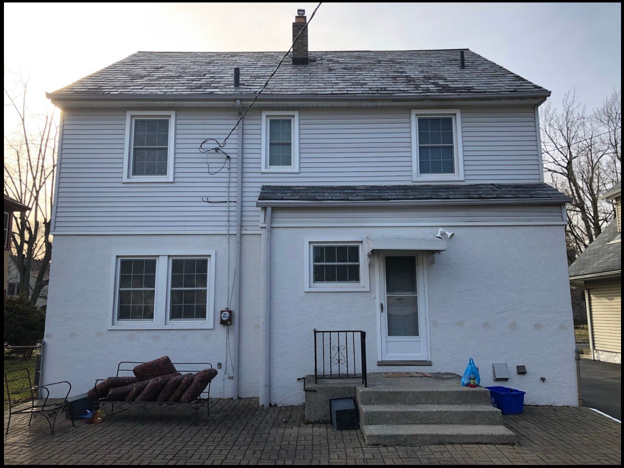
110 S. Stanwood Rd. - Back (East)
