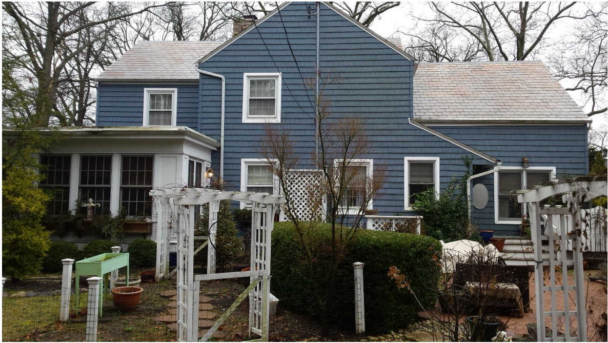
NORTH/ REAR VIEW
