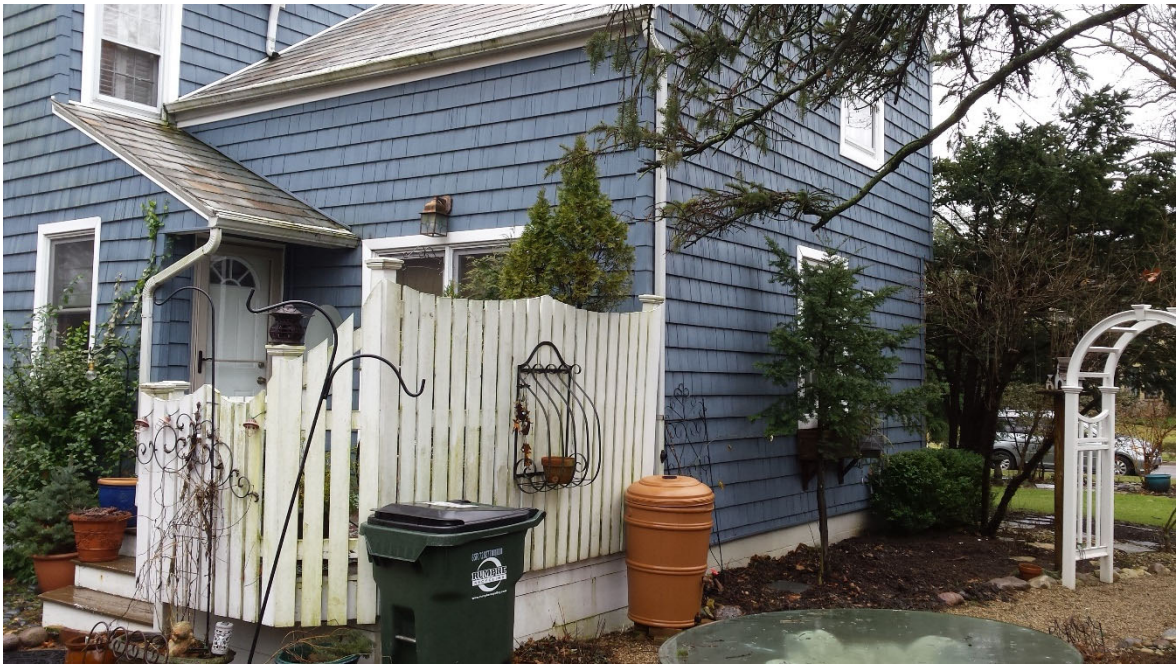
WEST/ LEFT SIDE VIEW
