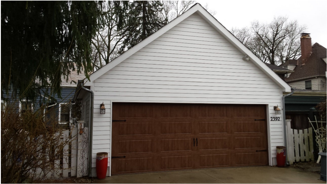
GARAGE – NORTH VIEW
