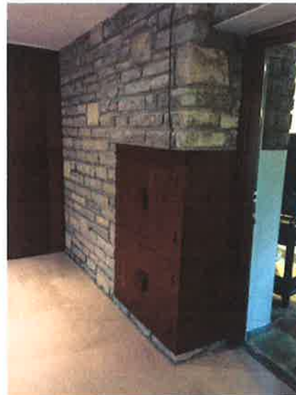
Interior NE corner of porch
