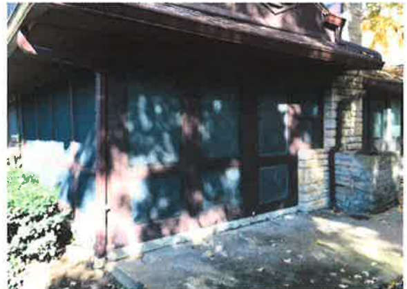
Corner view. Exterior door will be removed.
