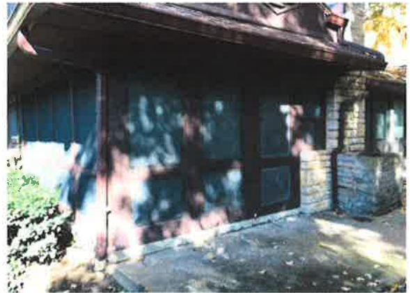
Corner view. Exterior door will be removed.
