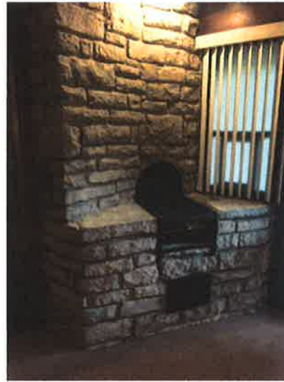
Interior SE corner of porch
