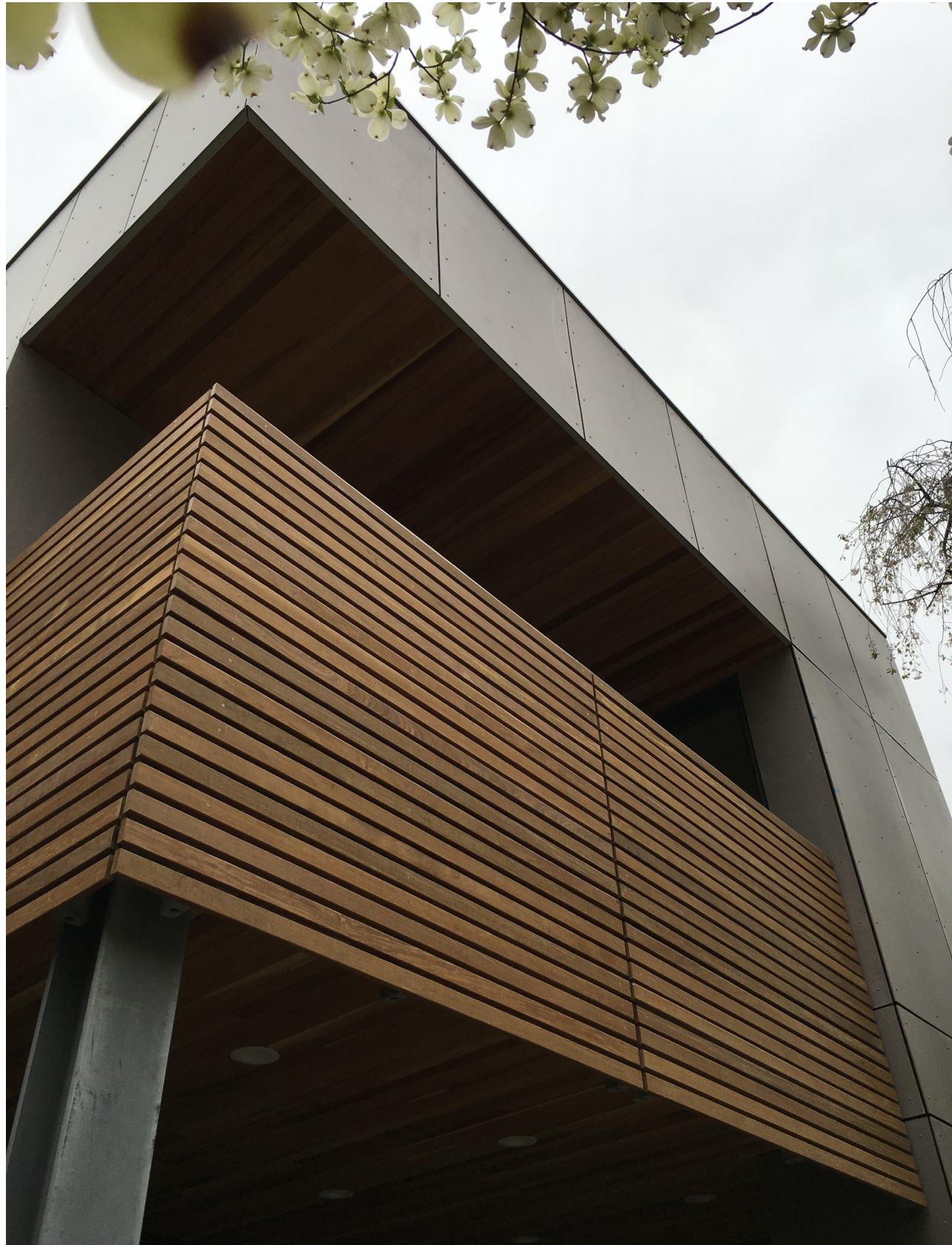
MATERIAL PRECEDENT - CEMENT PANEL SIDING
