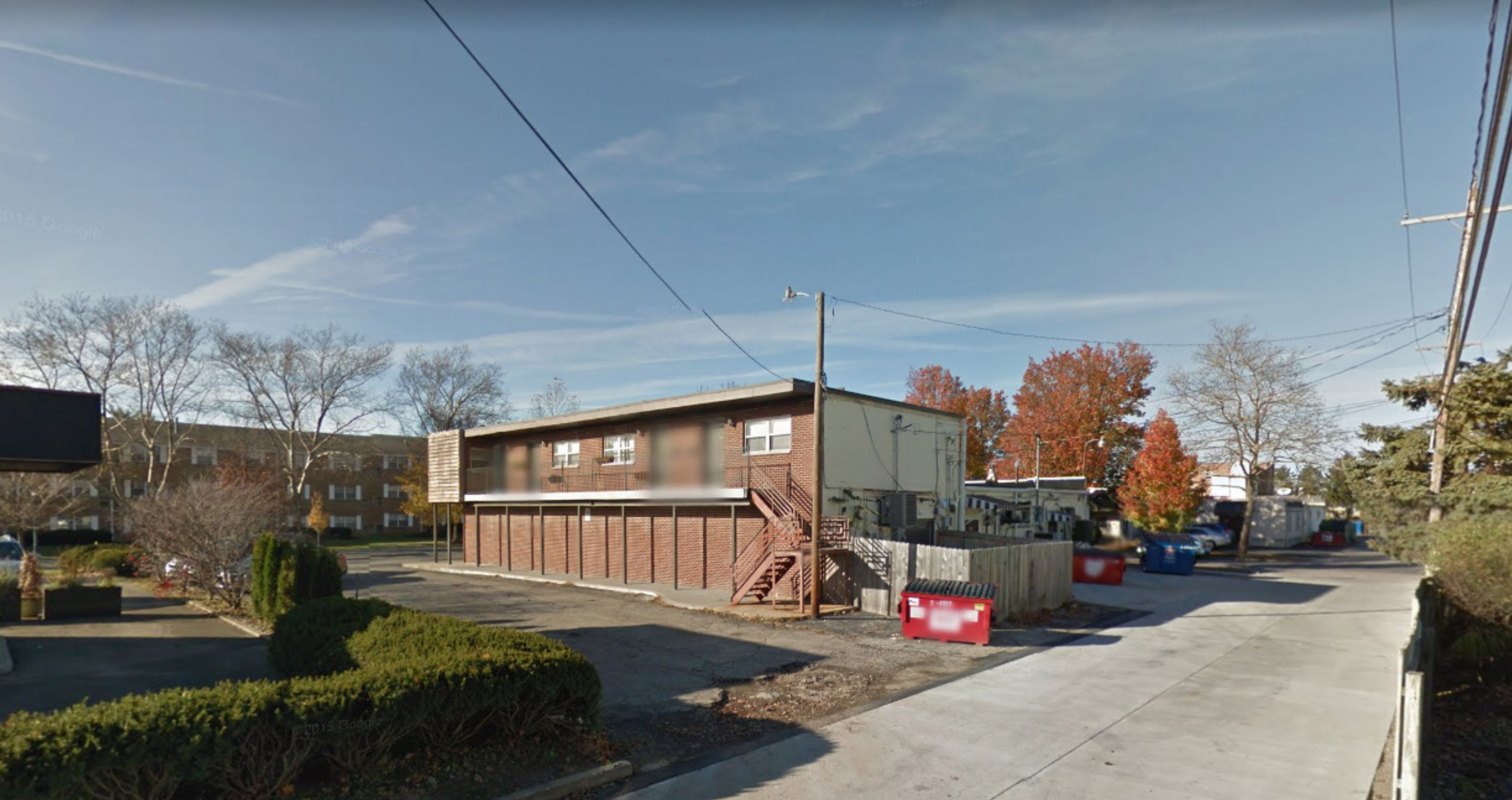
EXISTING ALLEY VIEW
