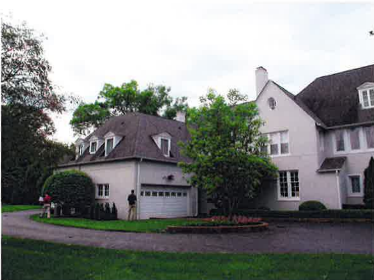
Photos of Existing North Side of Residence
