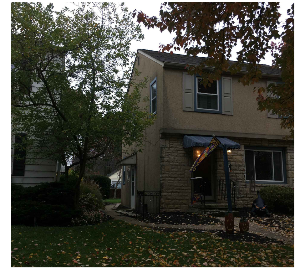
EXISTING SOUTH EAST CORNER
