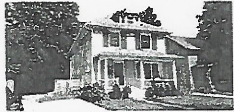
APPARENT ENCROACHMENTS: NONE.
