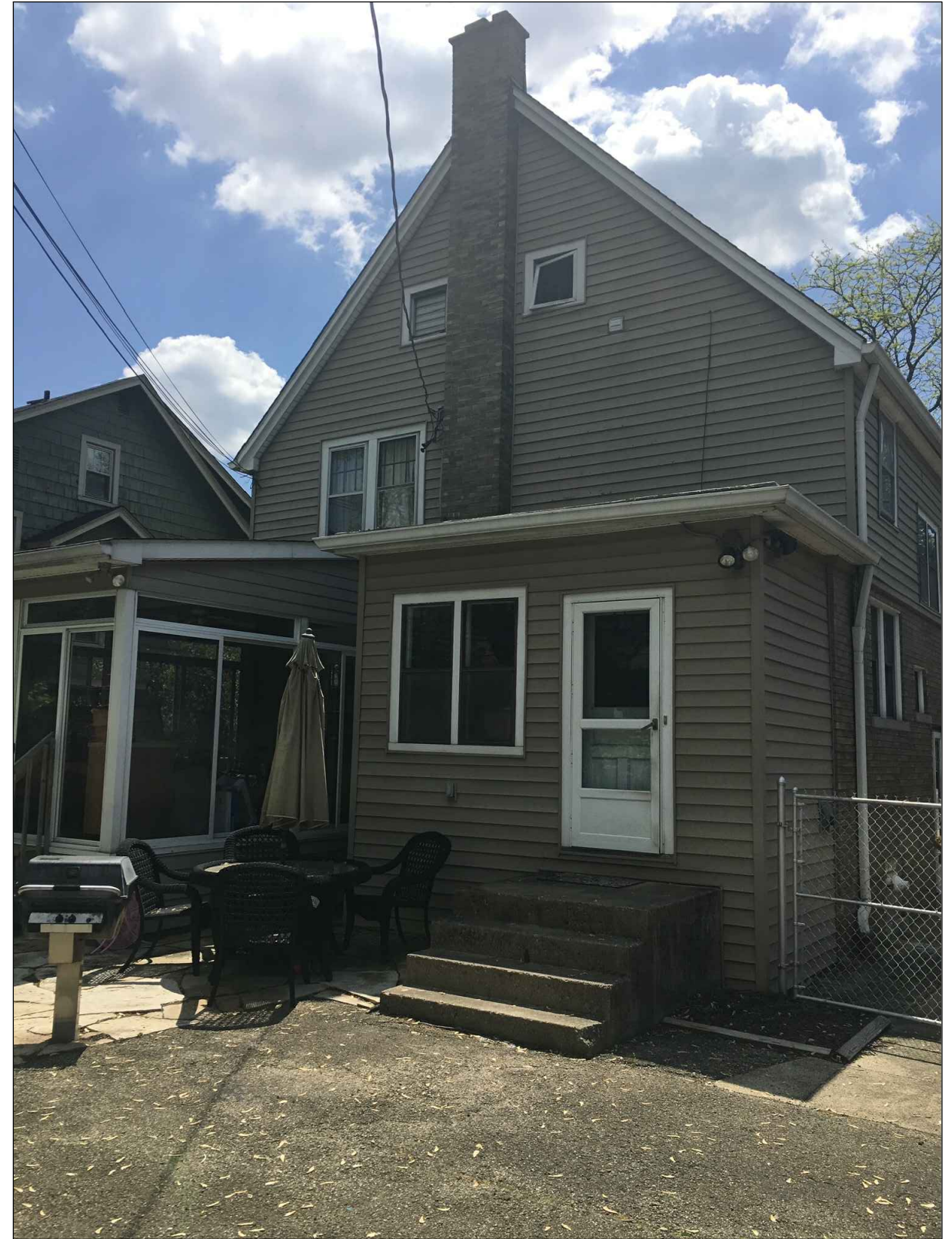
REAR FROM NORTHWEST
