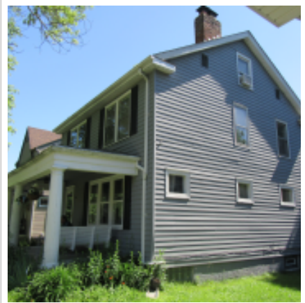
South Elevation Photo Mar 10, 2020
