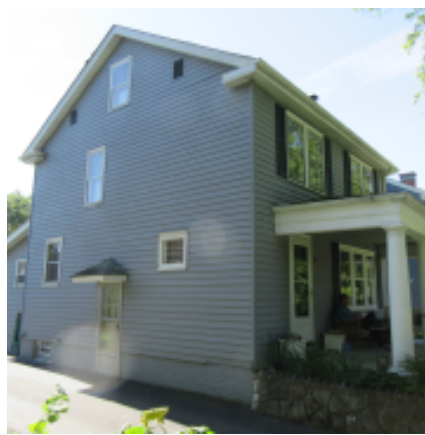
North Elevation Photo Mar 10, 2020
