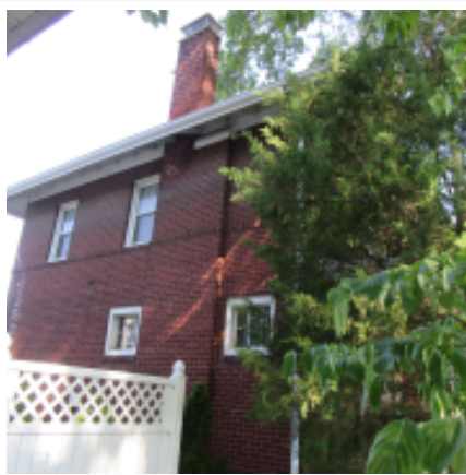
South Elevation Mar 10, 2020
