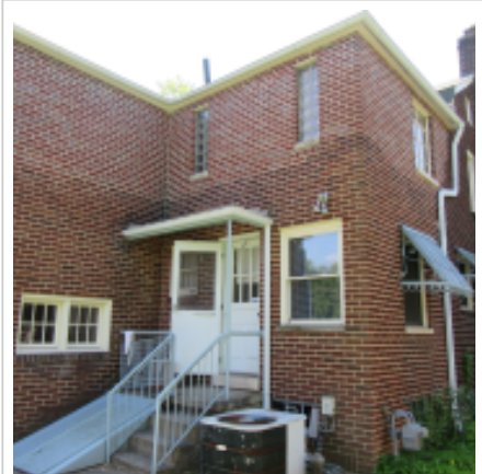
West Elevation Photo Mar 10, 2020
