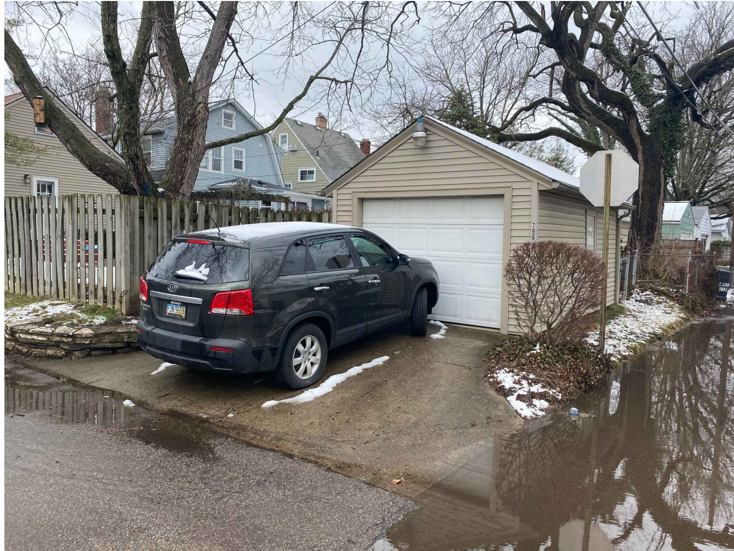
EXISTING GARAGE FROM SOUTHEAST
