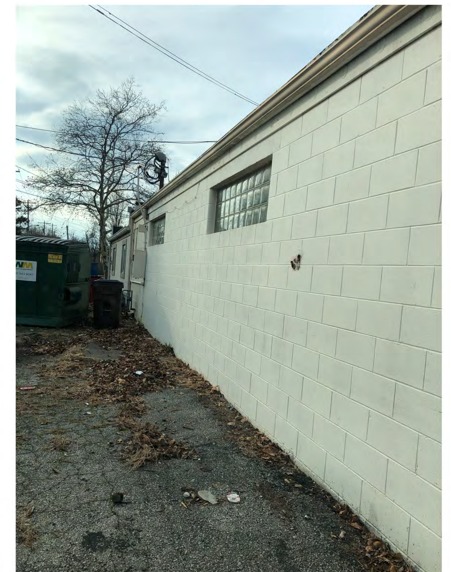
EXISTING WEST ELEVATION (REAR)
