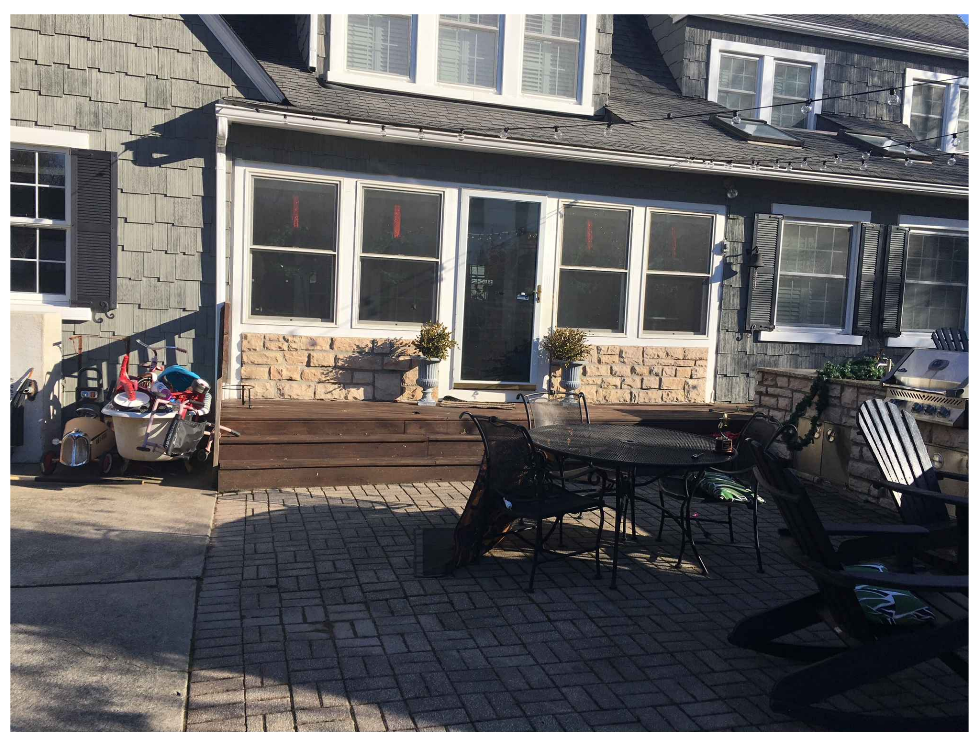
PORCH ENCLOSURE AND PATIO TO BE REMOVED
