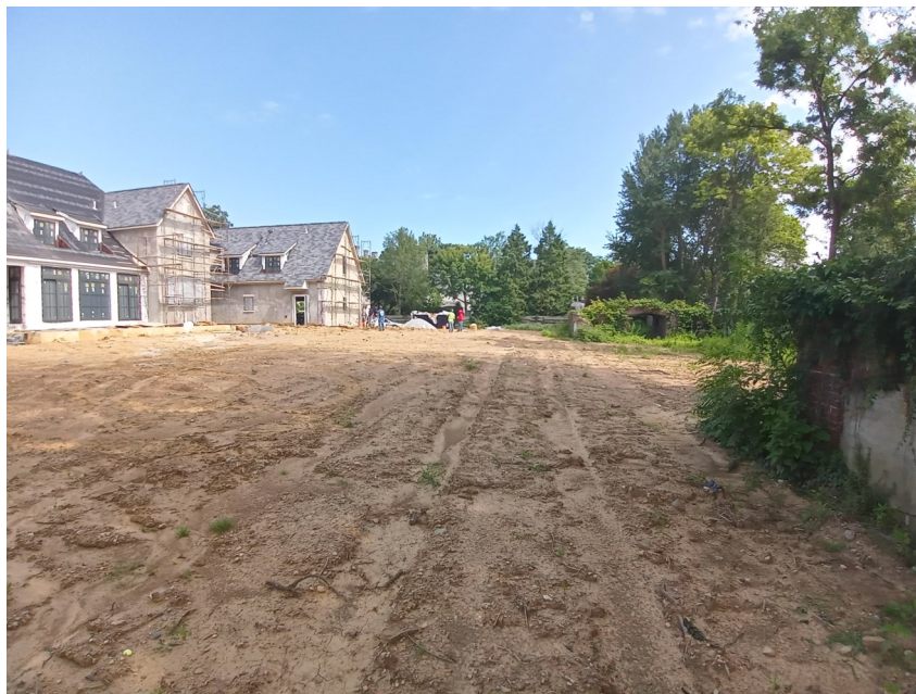
View from the South side looking North at proposed location of Pool House and Pool.
