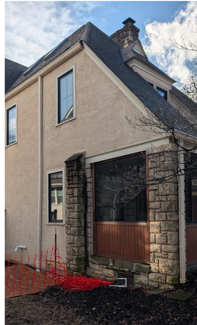
FRONT PORCH - EAST SIDE
