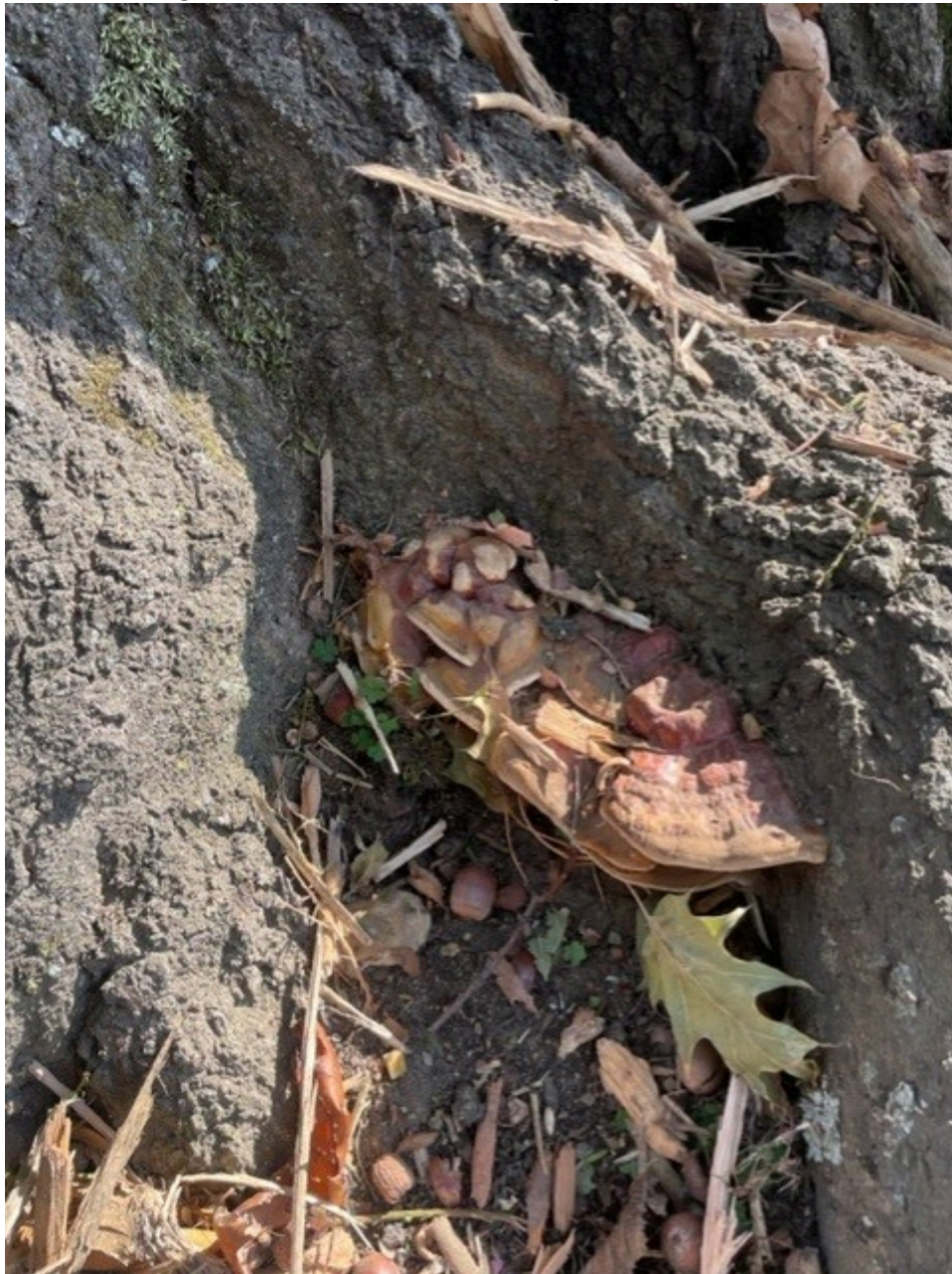
Below are images taken of the buttress root systems of three Red oak trees on SW corner of home
