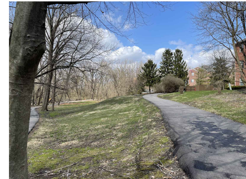
'BUMP' TO BE REGRADED AND AREA TO BE FILLED IN.
