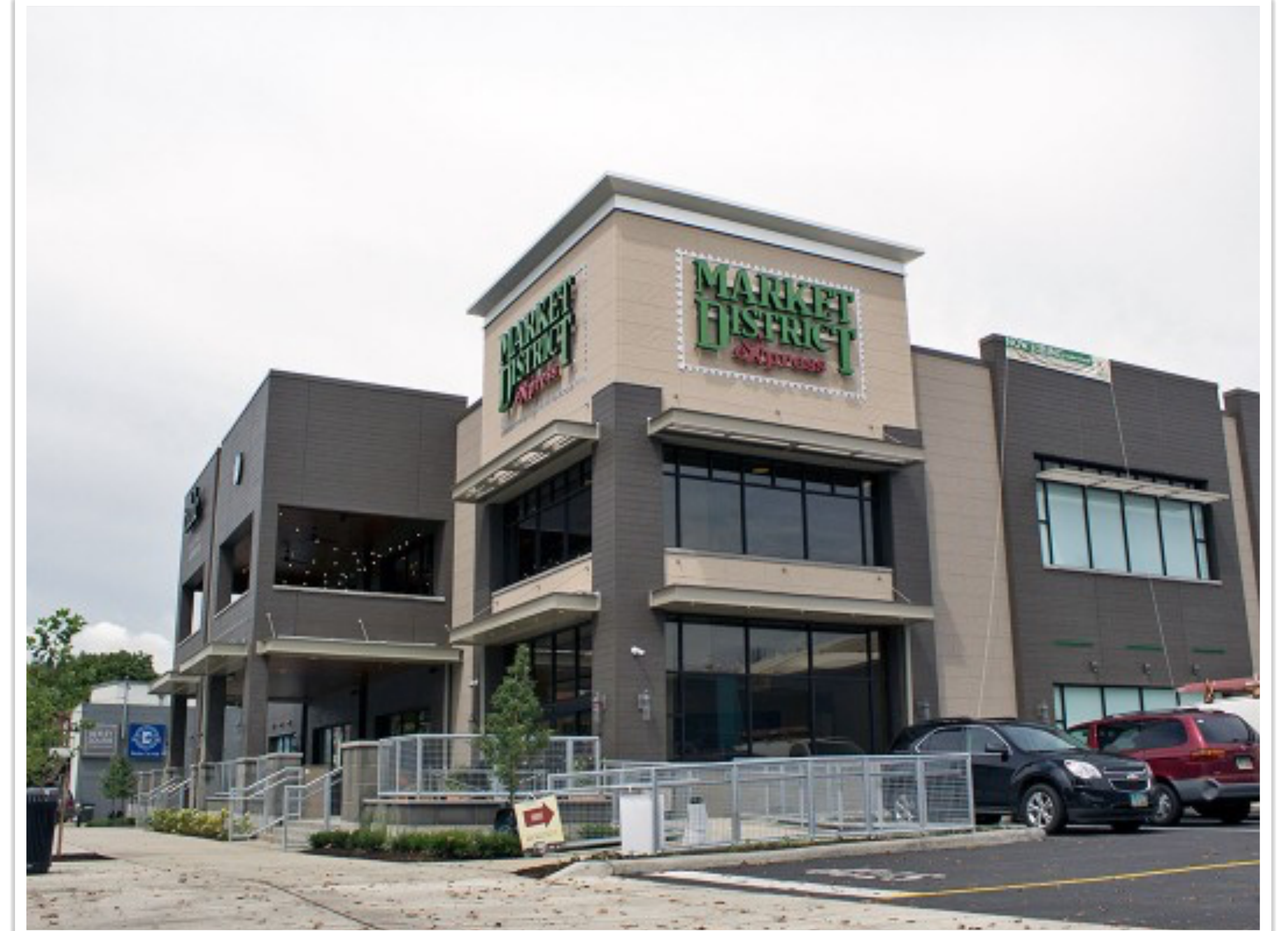
City Hall Site: Now
