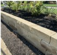
RETAINING WALL 6" LIMESTONE
