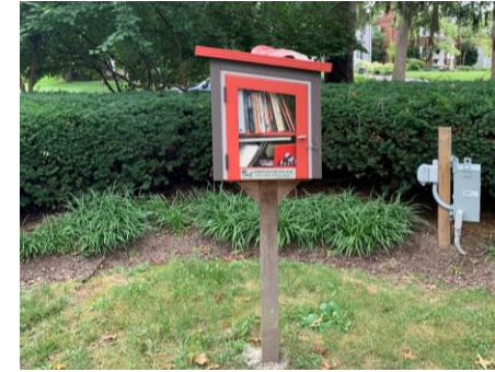
1 – Free Little Library and Electrical Service
