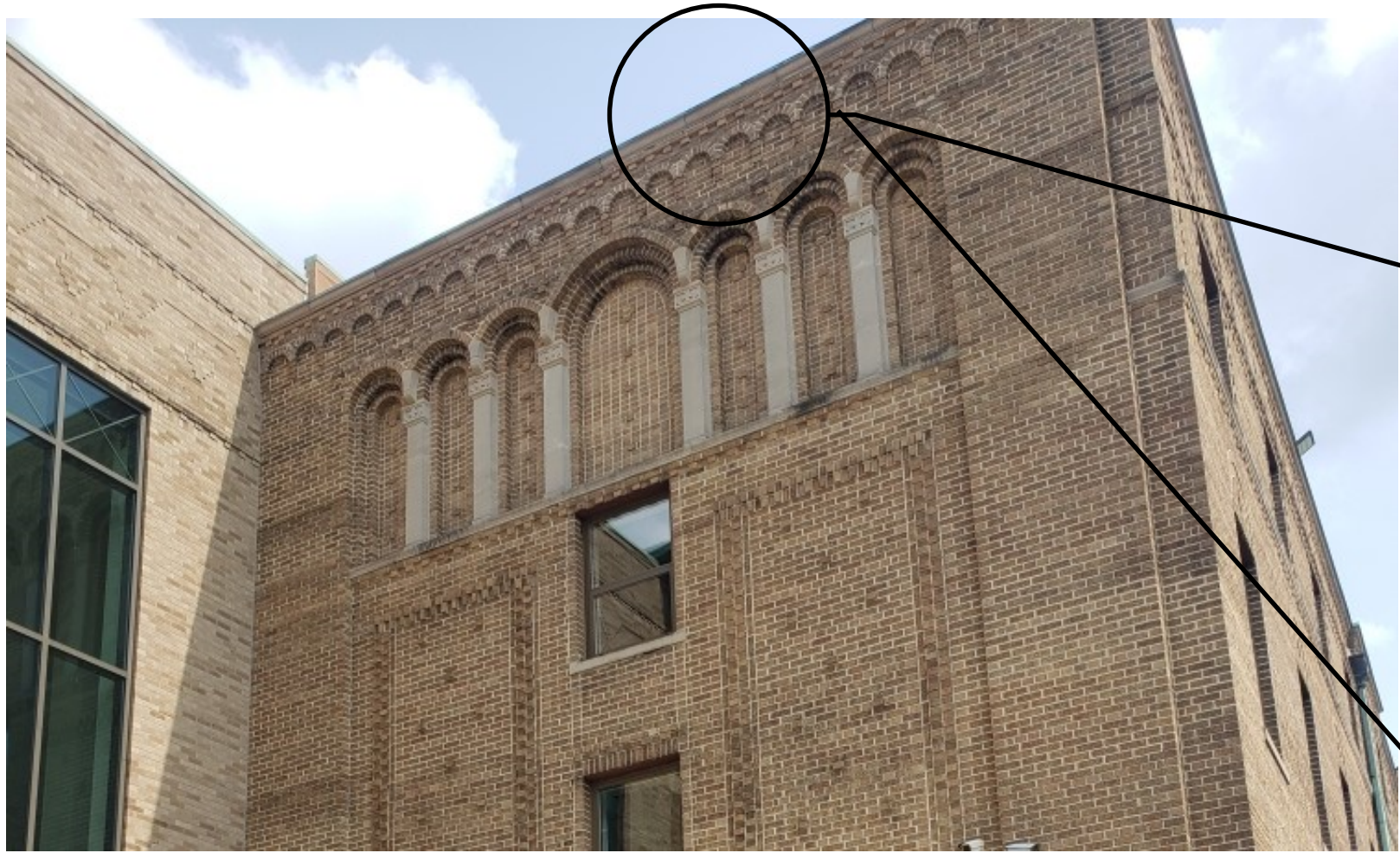
New brick arched cornice with limestone banding of the building will match the look and materiality of the existing school and convocation center. This will be continuous around the building.
