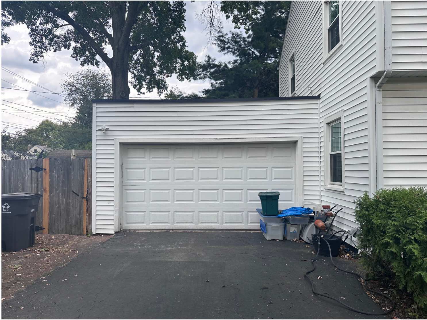
SOUTH FACADE - EXISTING
