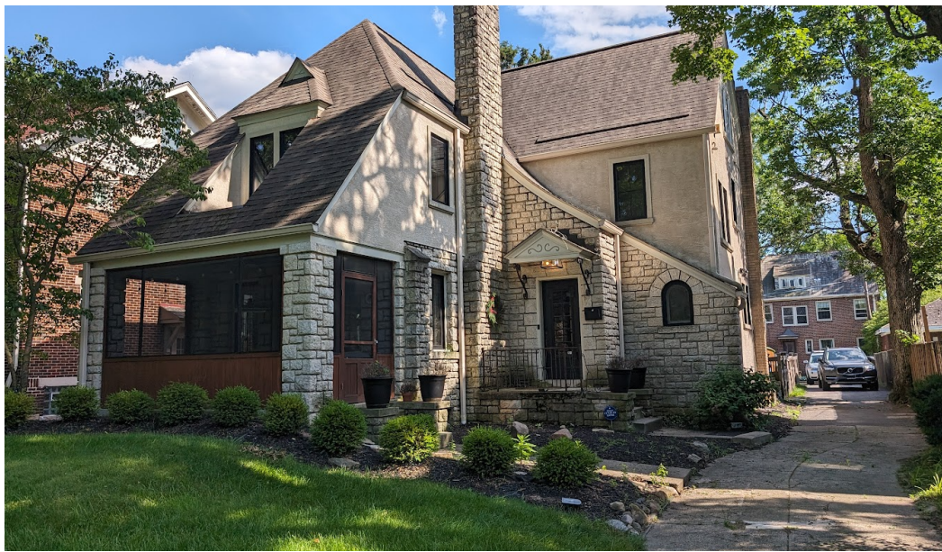
North Facade (Broad Street)
