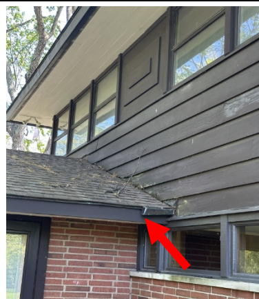
Exterior framing and downspout at west
