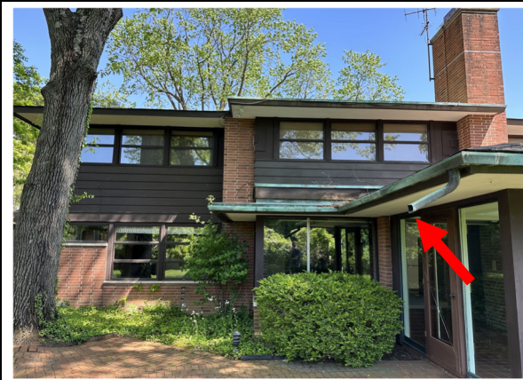
Gutter downspout at south side
