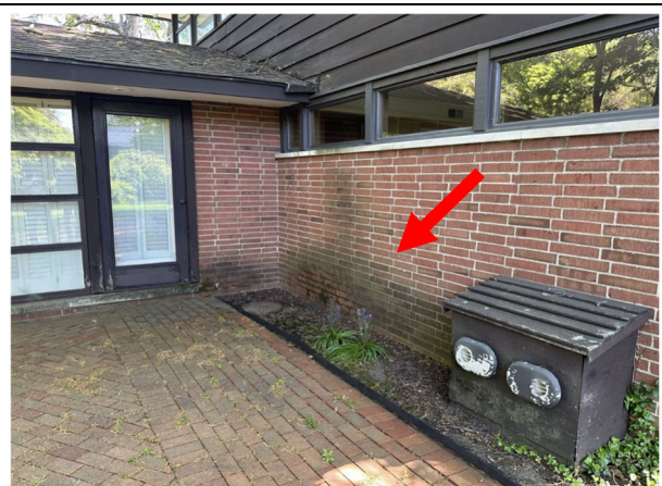
Exterior grade at west side
