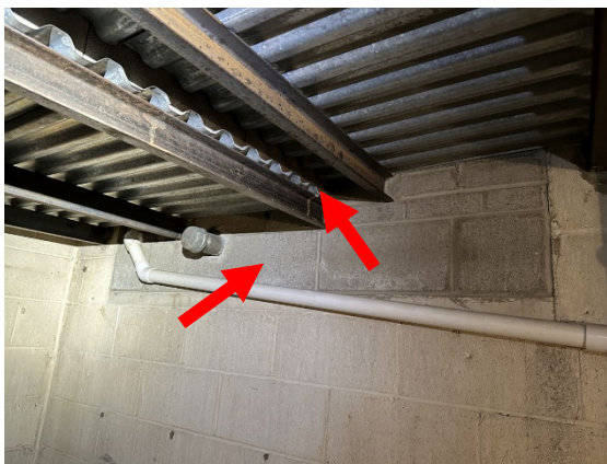
Window well infill and water mitigation framing
