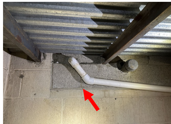
Window well infill and water mitigation framing
