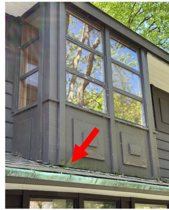
Exterior framing at north low roof
