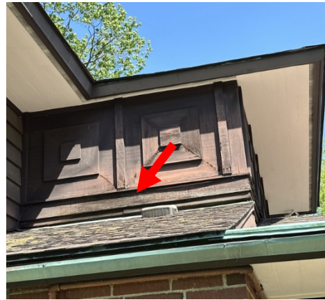
Exterior framing at south low roof
