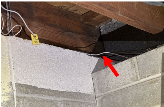
Rim board water infiltration
