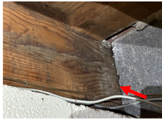
Rim board water infiltration at corner
