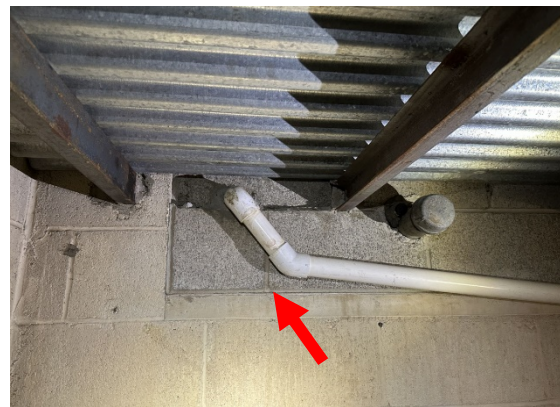
Window well infill and water mitigation framing
