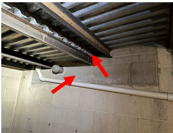
Window well infill and water mitigation framing
