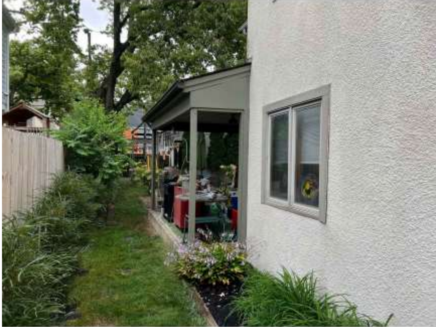
SOUTHWEST PORCH TO BE ENCLOSED
