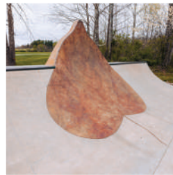
Nashville, IN - Acid Staining | Scoring, Custom Form
