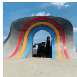
New Albany, IN - Flowpark Entrance | Scoring | Polymer Concrete Staining
