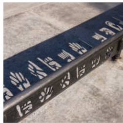
Indianapolis, IN - ASL rail | Decorative Welding | Steel Fabrication
