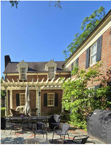
North Facades of Existing Residence
