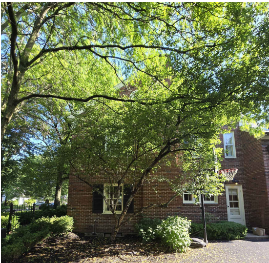
West Portion of South Facade of Existing Residence
