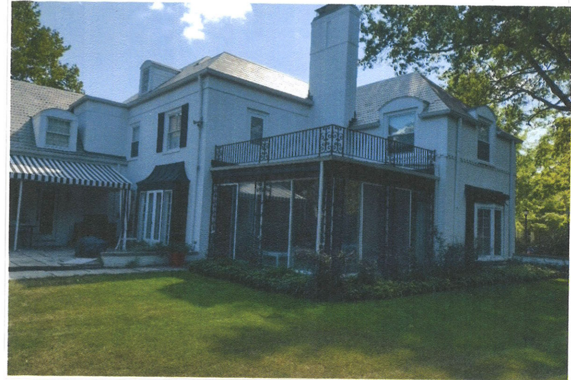
PORCH & PATIO PHOTO
