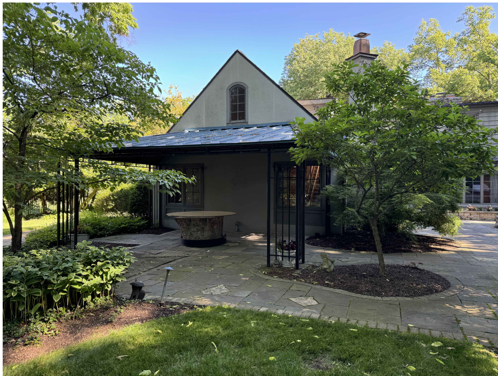
C EXTERIOR PHOTO - SOUTH ELEVATION SCALE: NTS
