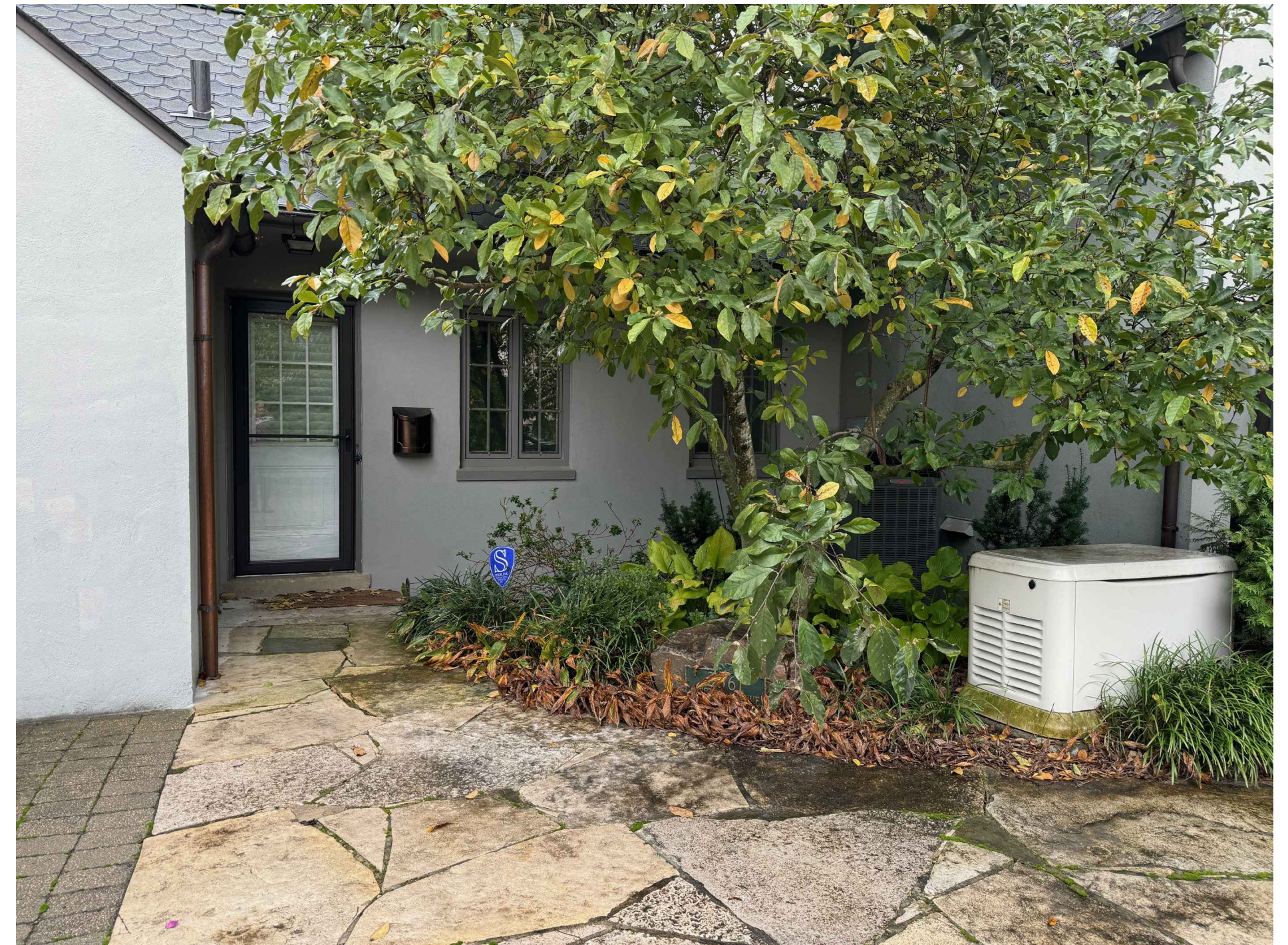
B REFUSE ENCLOSURE AREA - LOOKING EAST
