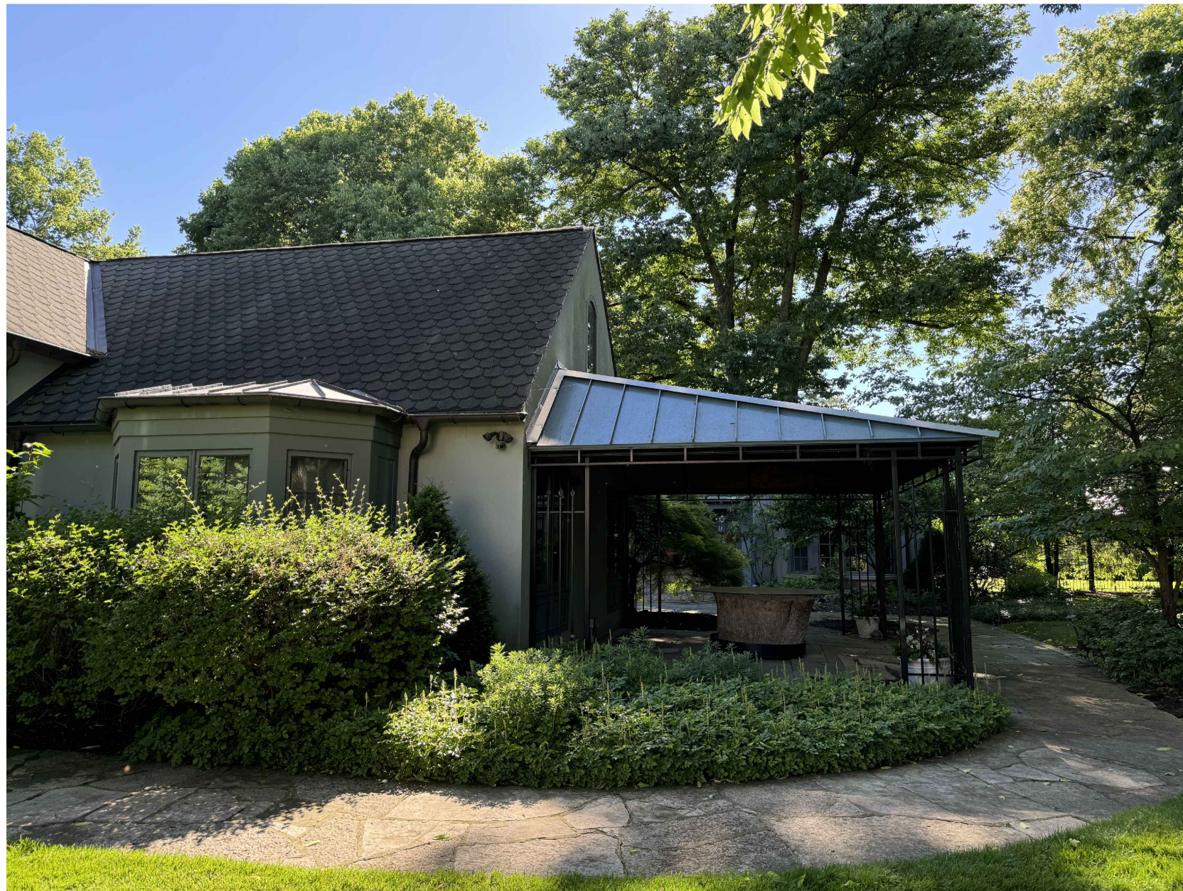
A EXTERIOR PHOTO - WEST ELEVATION SCALE: NTS
