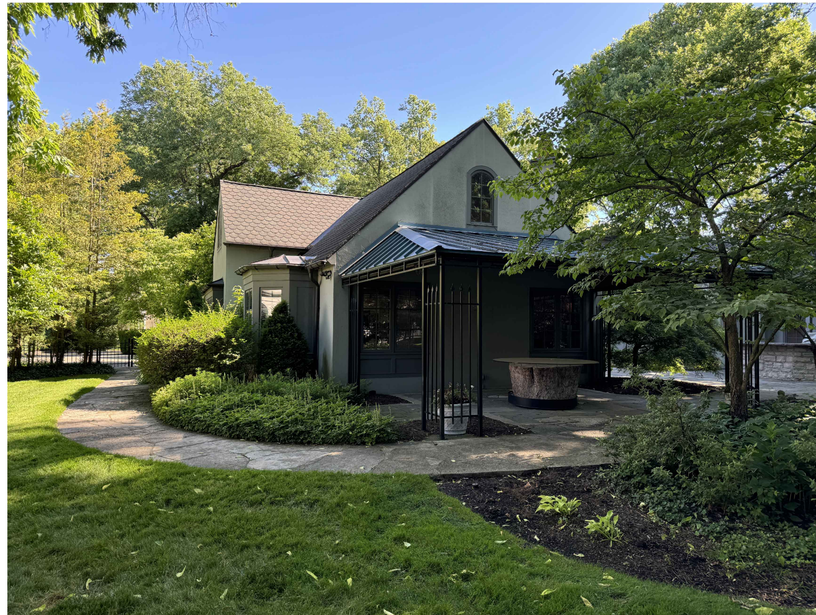
B EXTERIOR PHOTO - SOUTHWEST ELEVATION SCALE: NTS
